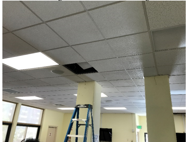
Third Floor Suspended Ceilings
