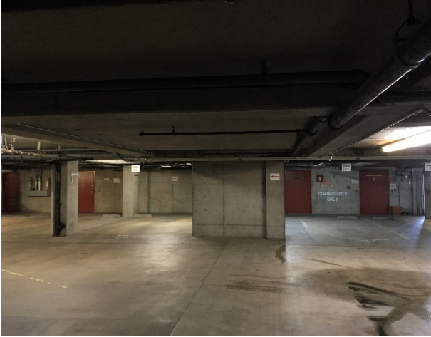
Building Basement & MEP Bracing
