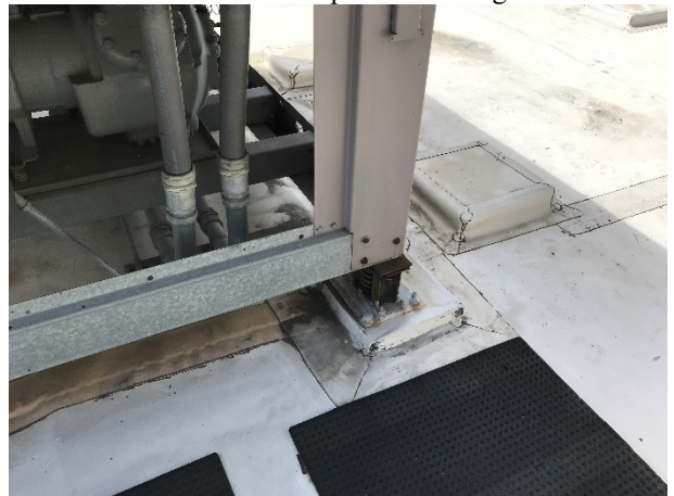
Third Floor Roof mounted equipment anchorage
