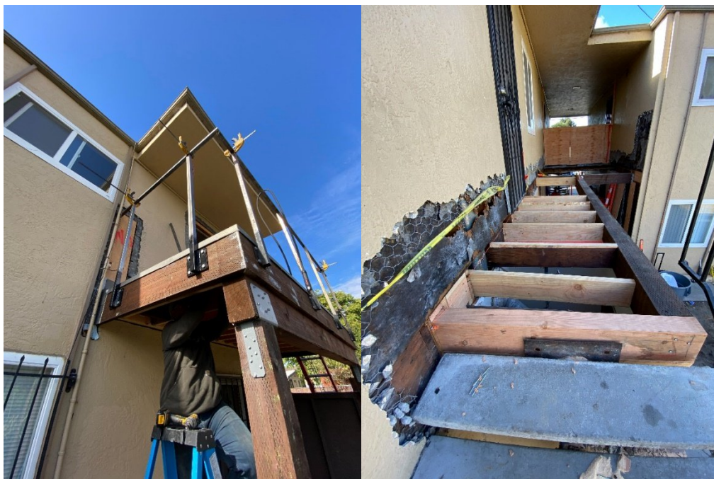
9329 Sunnyside Deck Dry Rot Repairs
